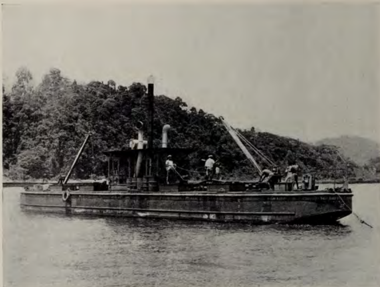
PALM OIL TANK BARGE.
