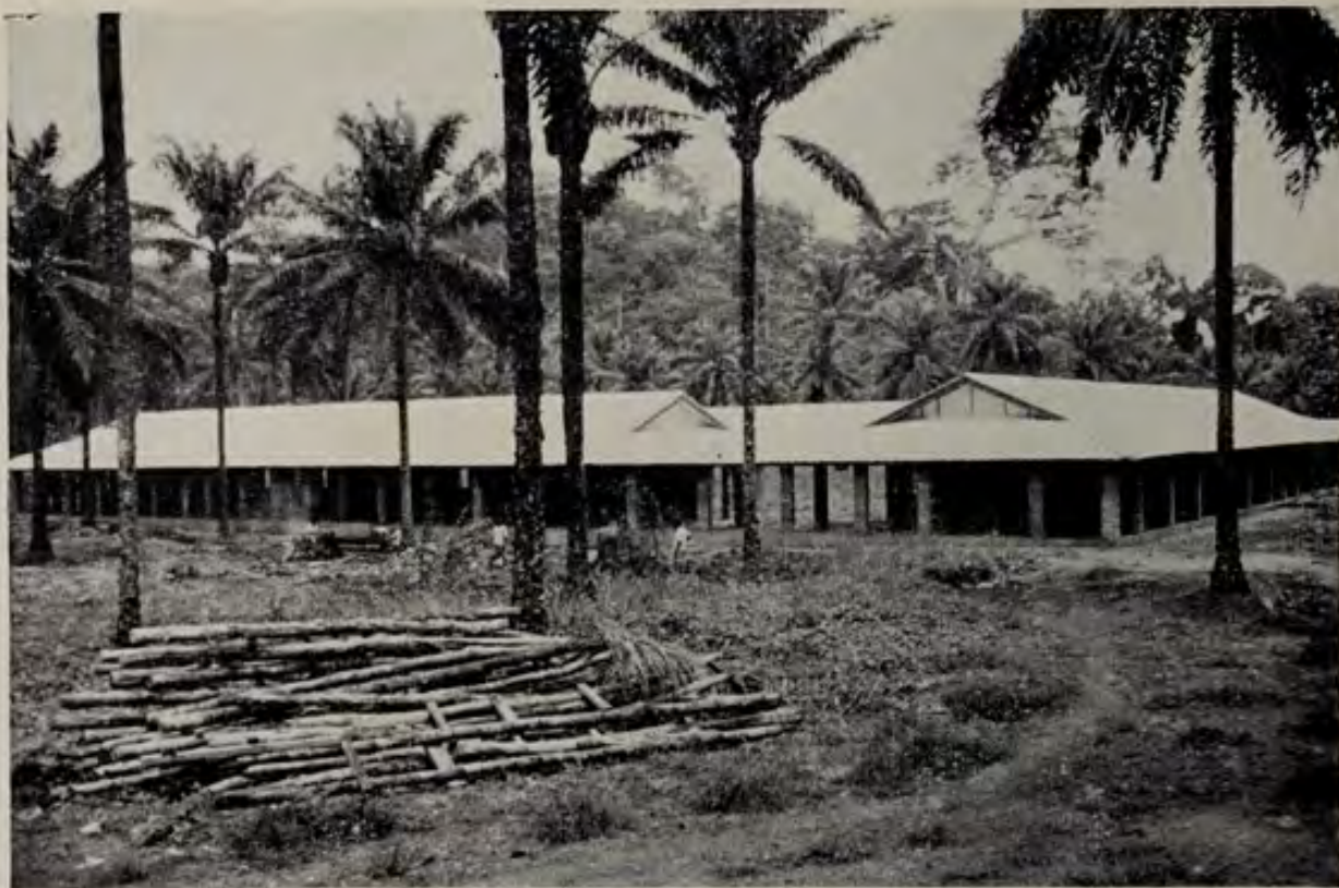
BOTA HOSPITAL (under construction).
