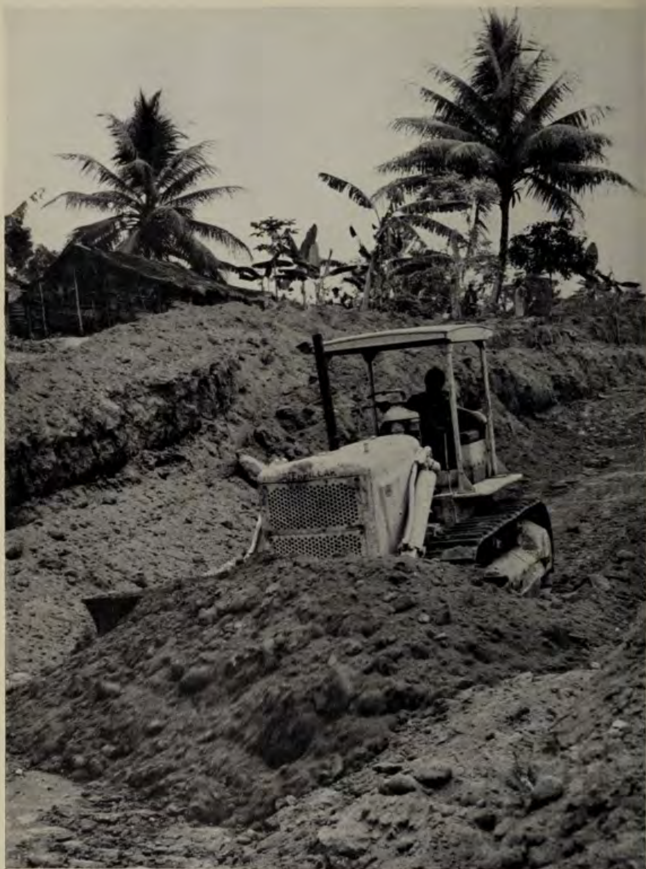
Road construction: remaking the Victoria-Kumba Road
