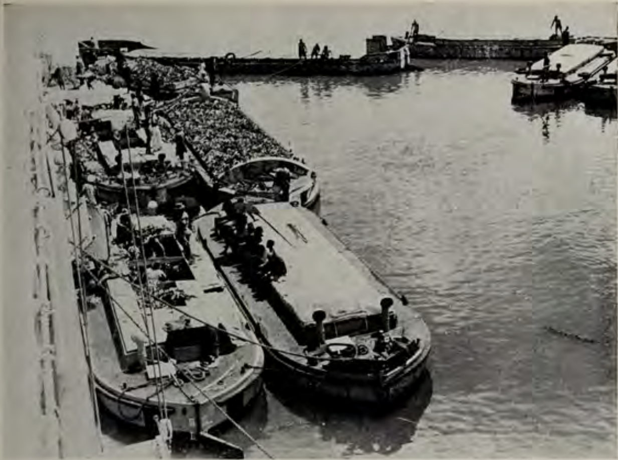
LOADING OVERSIDE FROM LIGHTERS.
