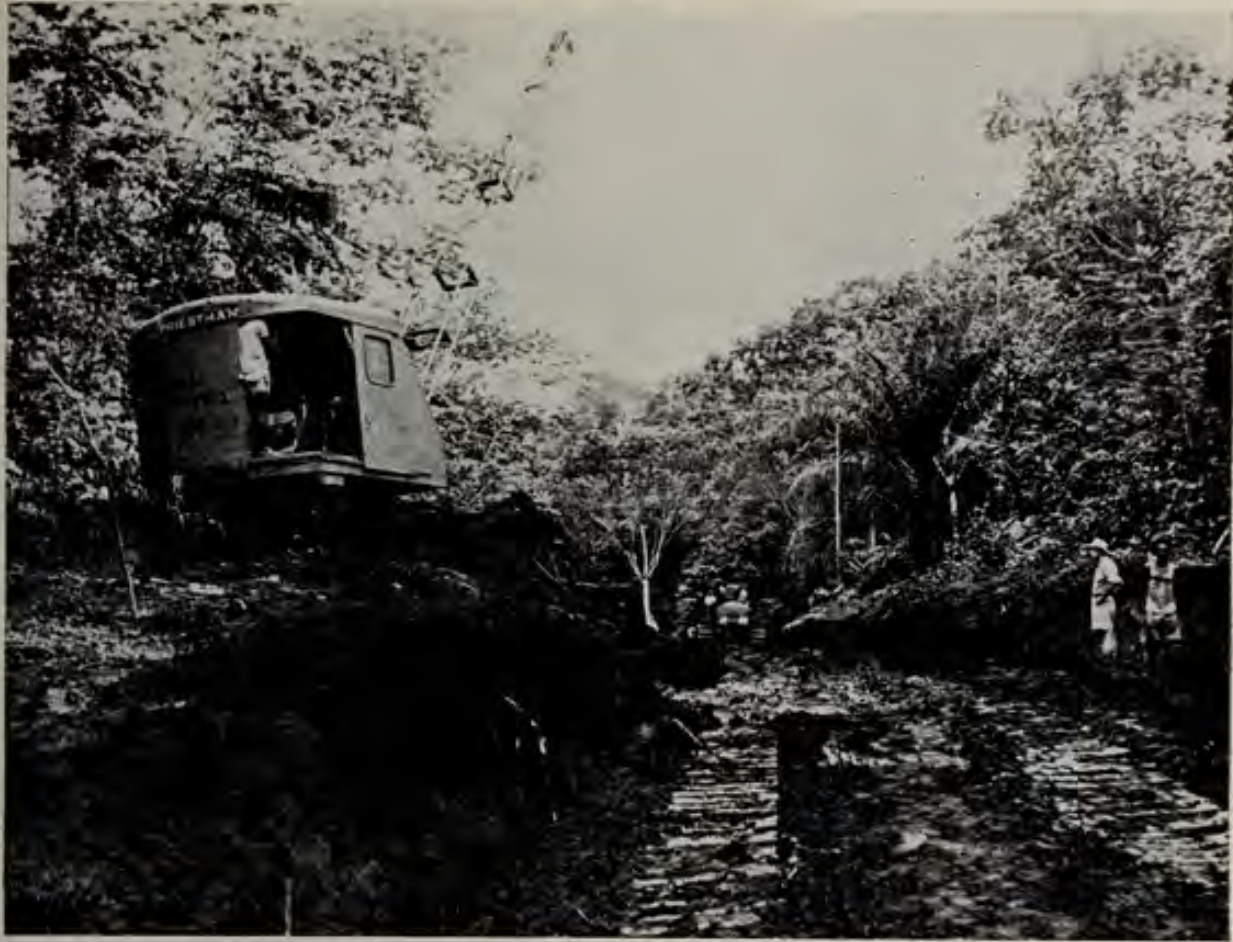
EXCAVATIONS FOR ROAD.
