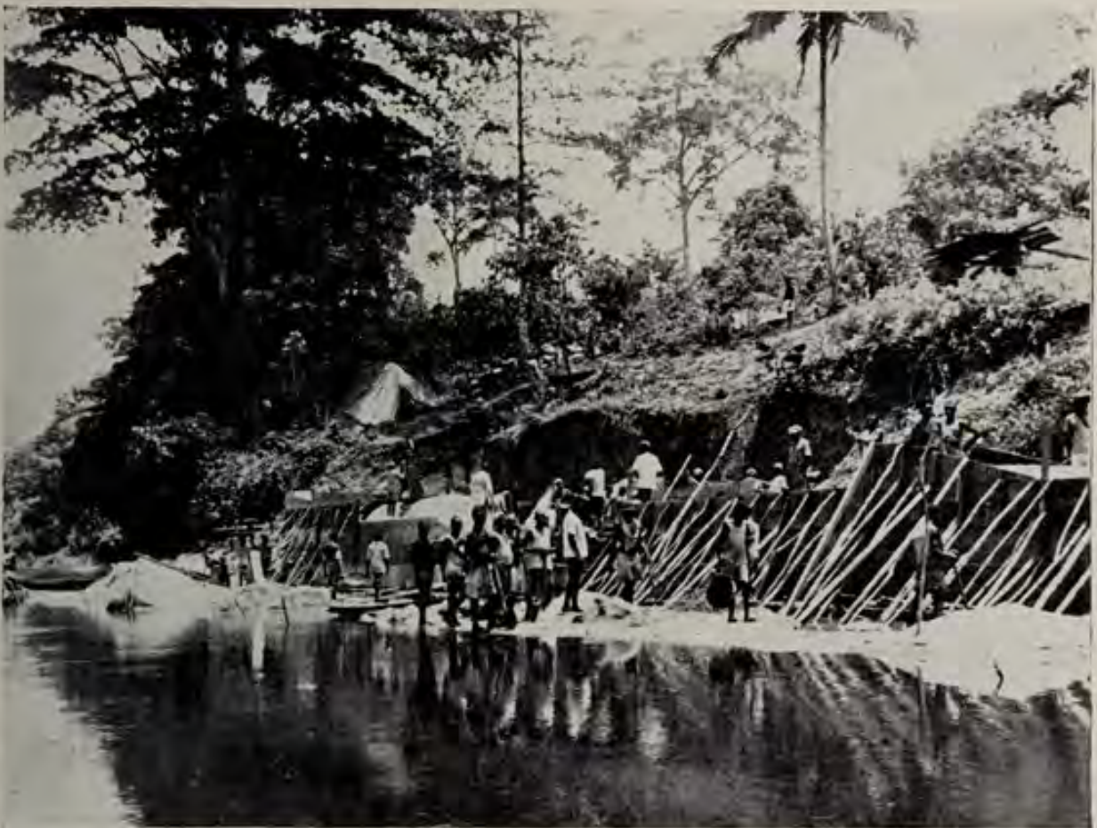
MUNGO FALLS WHARF (under construction).
