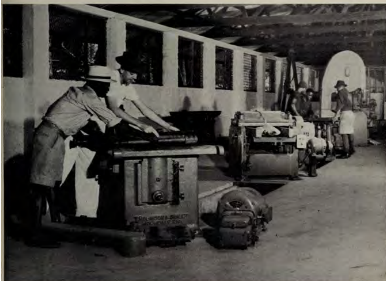
Ombe River Government Trade Centre—Machinery being installed
