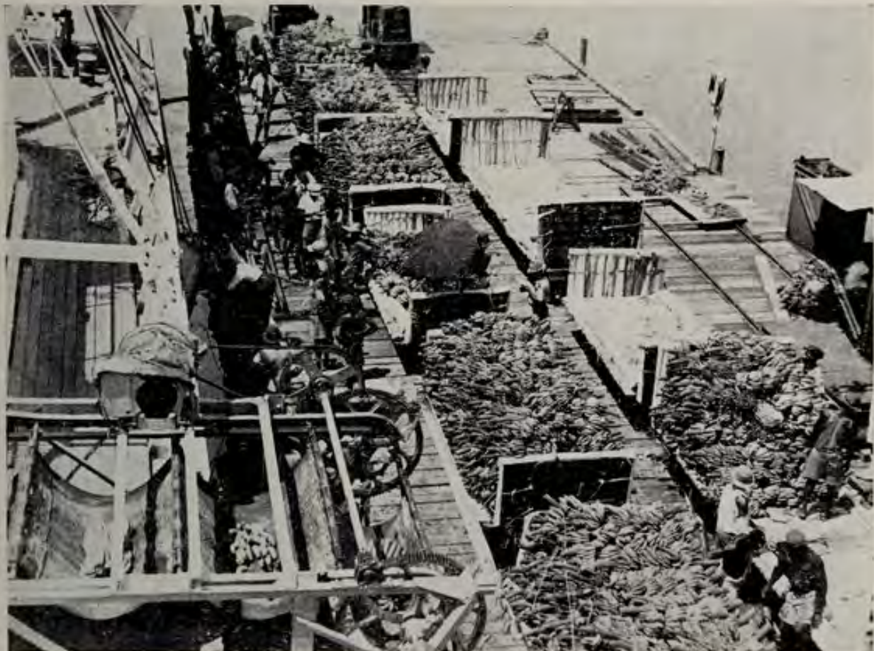
LOADING BY ELEVATOR FROM RAILWAY TRUCKS, TIKO.
