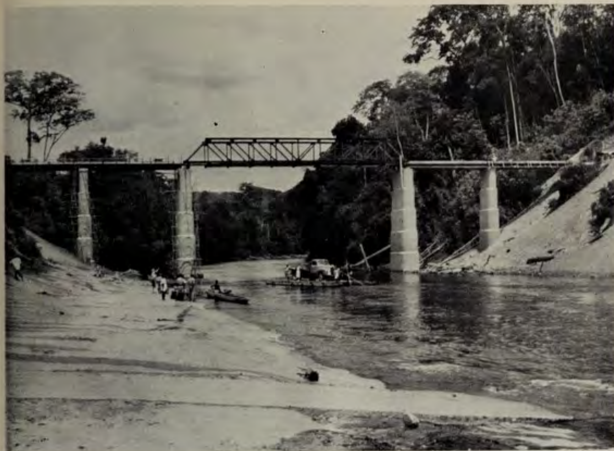
The Munaiya Bridge nearing completion
